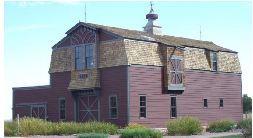
This 1888 Barn, located at Arrowhead Park, has lasted generations and will continue to last because of careful and continual preservation
